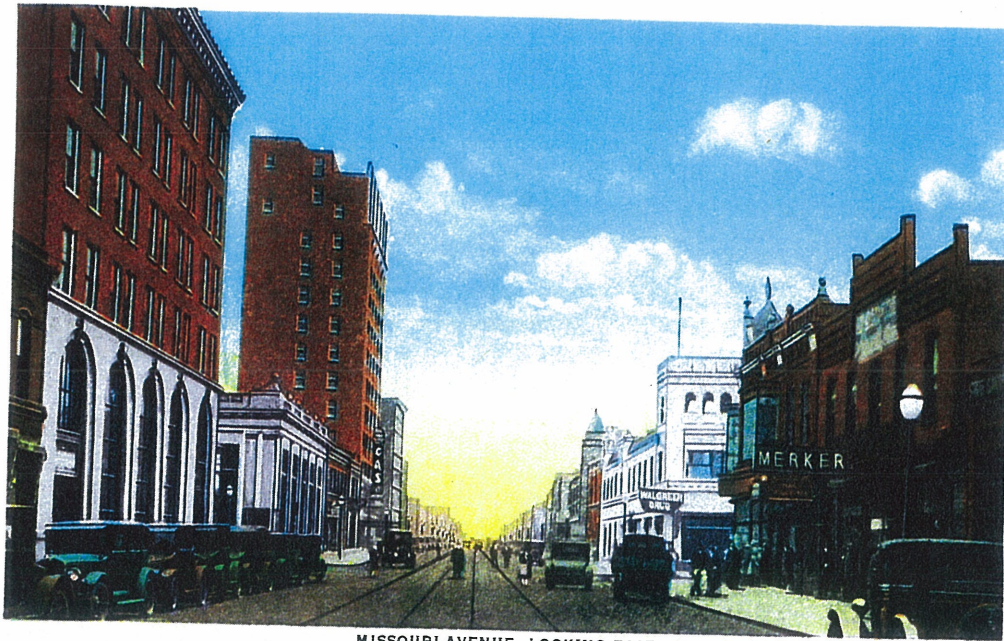
MISSOURI AVENUE, LOOKING EAST
